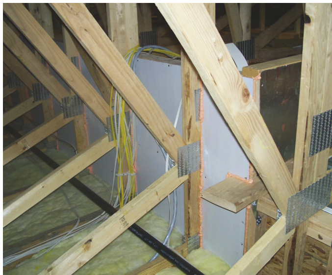
IMAGE depicts a properly sealed air barrier at an attic knee wall.
